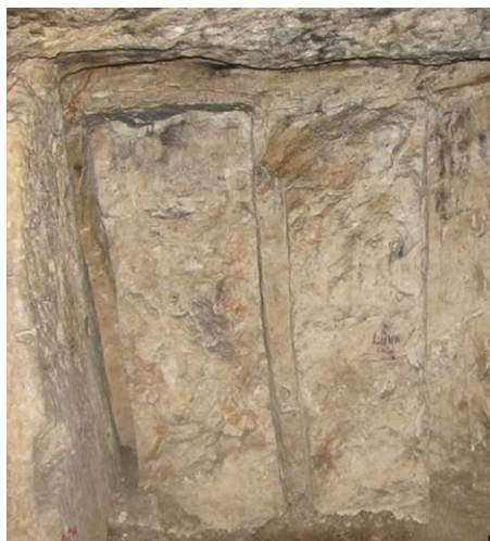
The channels for the wooden wedges can be clearly seen in this photo.
