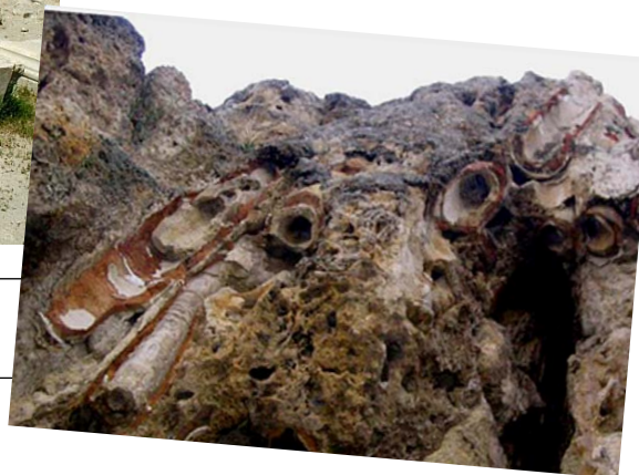
Evidence of high mineral content in terracotta pipes which carried the water about 5 miles to Laodicea.
